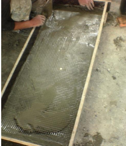
Fig 2: Placing the wiremesh
