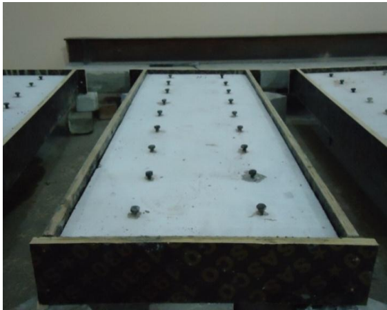
Fig.4: Placing the bolts to connect the ferrocement cover and repaired slabs
