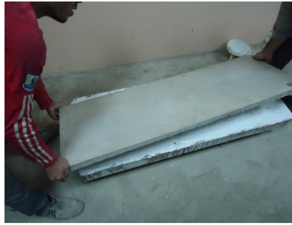
Fig.5: Placing the ferrocement cover connected to repaired slabs by epoxy
